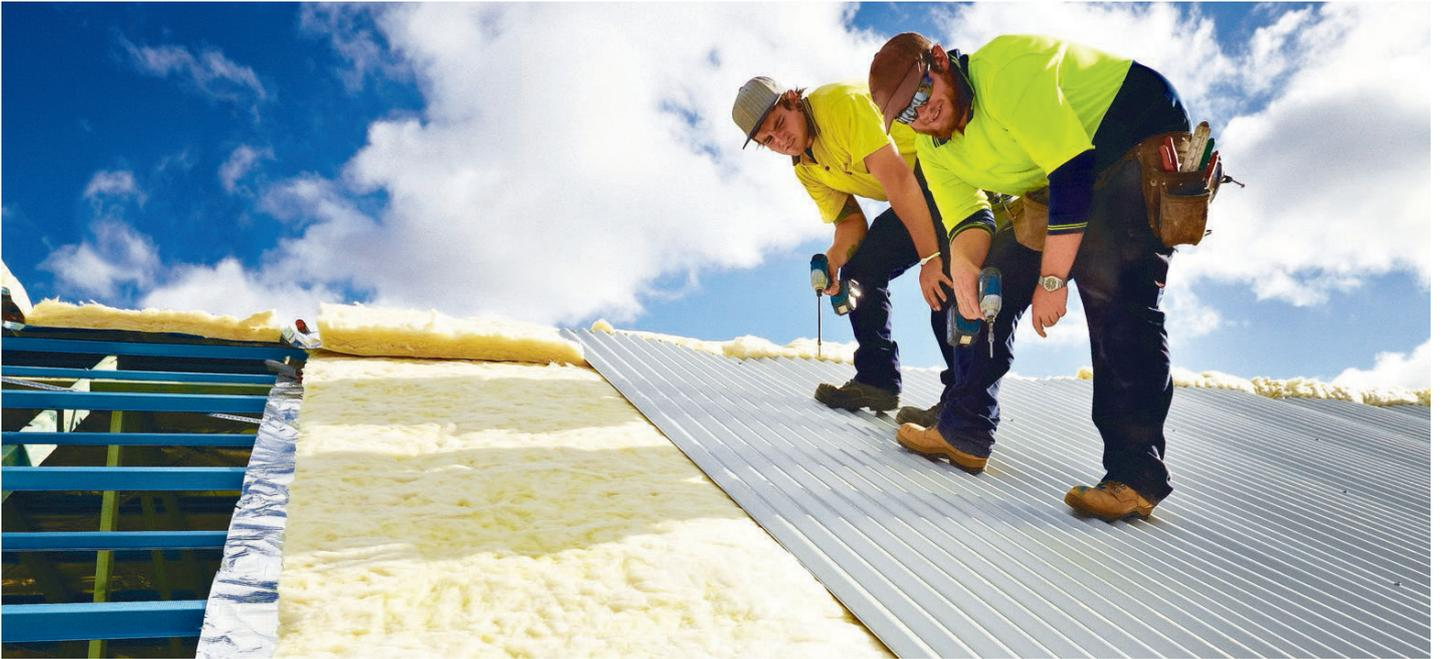
NCC 2022 requires metal roofs, under certain circumstances, to have a thermal break installed between the metal roof sheeting and the steel structure beneath it. This is to mitigate the effects that thermal bridging may have on the metal roof system.
