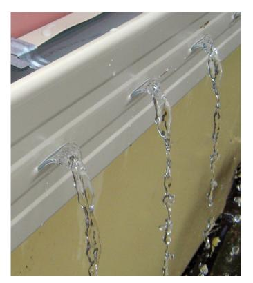
Typical overflow from slotted gutter. (Gutter shown is not available in all areas).
